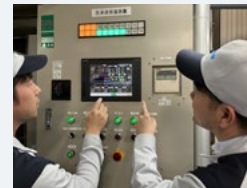
Checking for heat loss in real time
