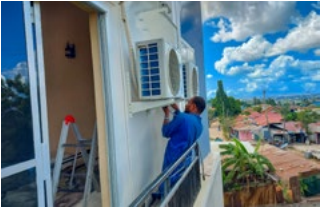
Installing an outdoor unit on a house
