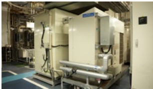
JIZAI HEAT installed at the Rinkai Factory
