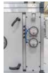
Fig 16: Magnehelic Gauge
