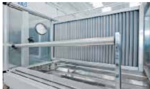
Fig 37: Steam Humidifier
