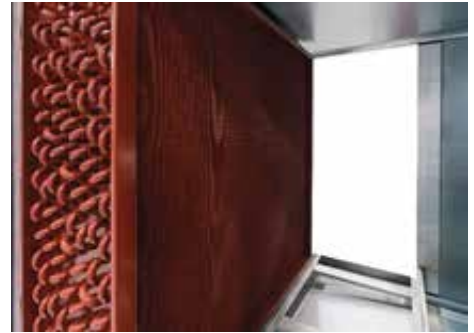
Fig 20: Coils with Herasite Coating
