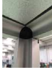
Fig 1: Internally Rounded Profile
