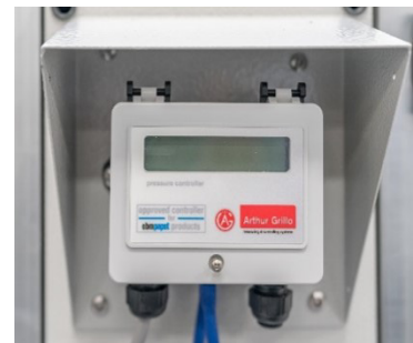
Fig 28: Airflow/Pressure LCD Controller
