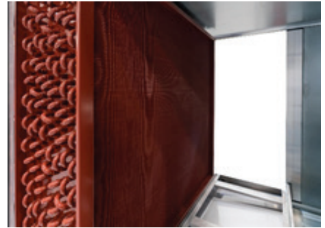
Fig 20: Coils with Herasite Coating
